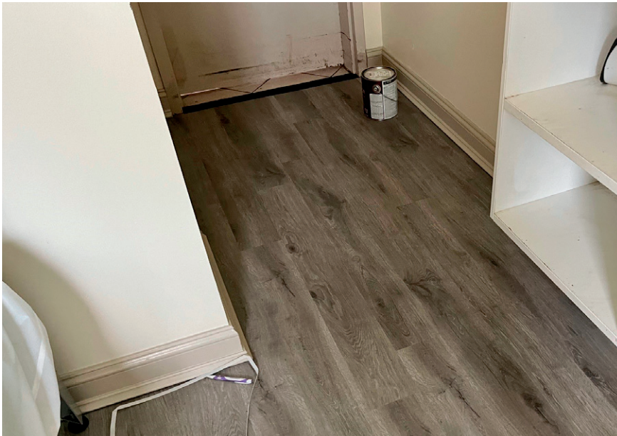
NEW FLOORING in the Large Family Room
