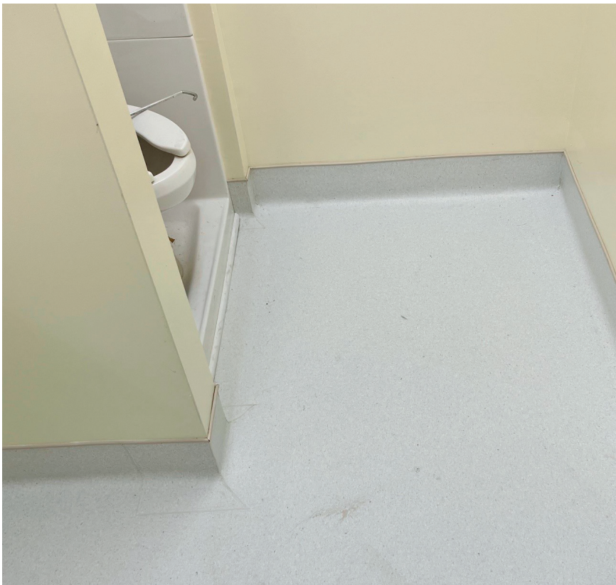
NEW FLOORING in the Bathroom/Shower
